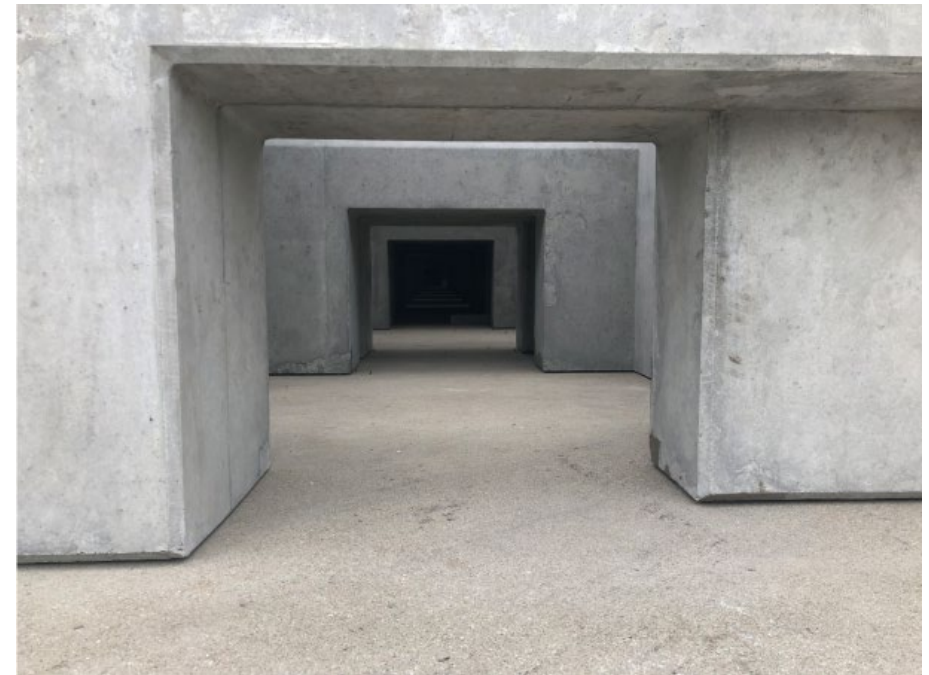
Internal vent channels within group of NUHOMS HSMs
