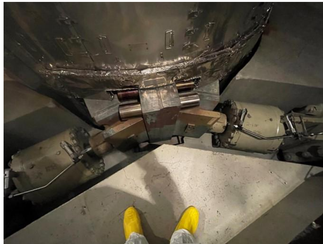
Large and Small Snubbers in Containment
