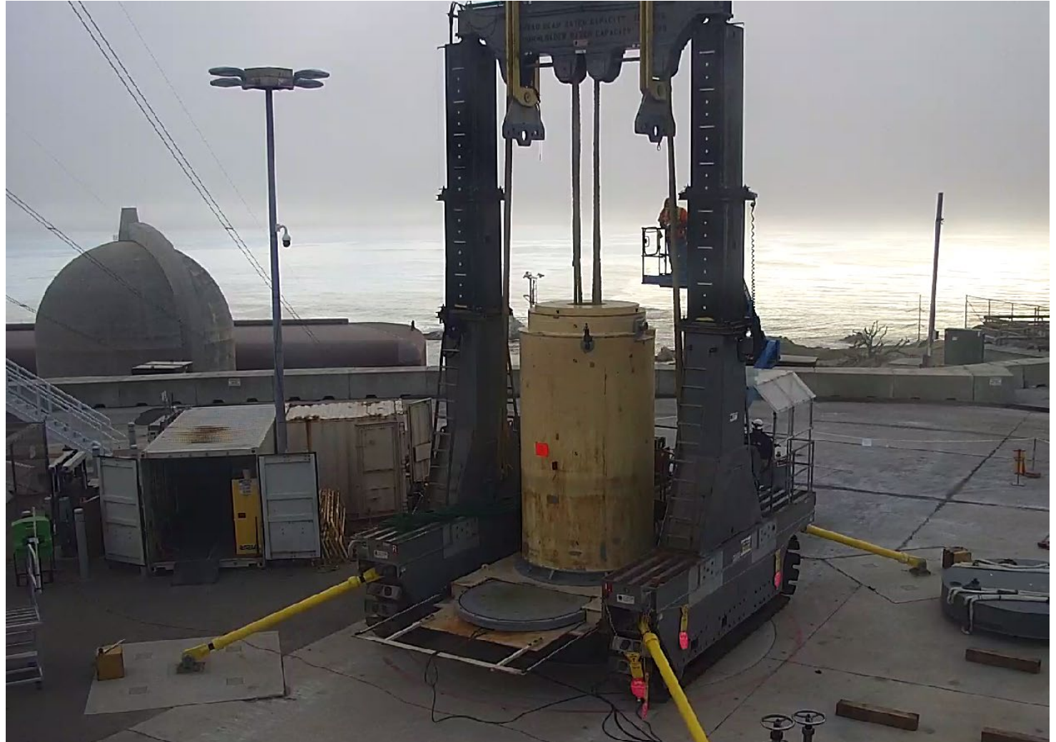
Transferring MPC from Transfer Cask to Storage Cask
