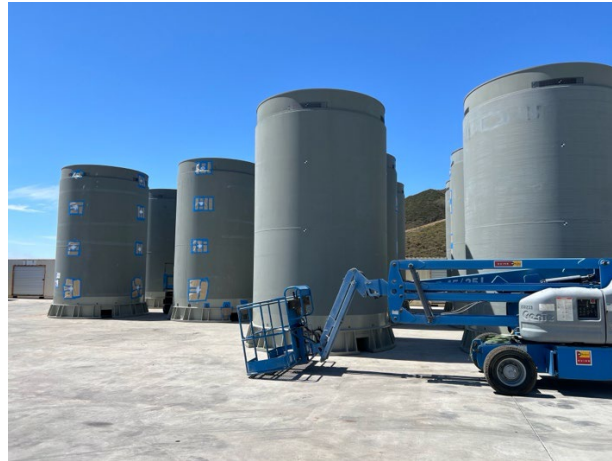
New Concrete/Steel Overpacks Awaiting Loading
