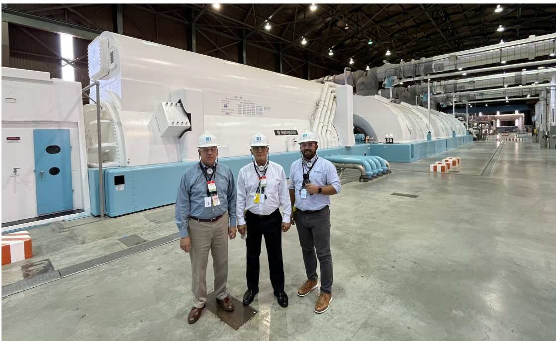
FFT and Mr. McBride at Unit 2 Main Generator
