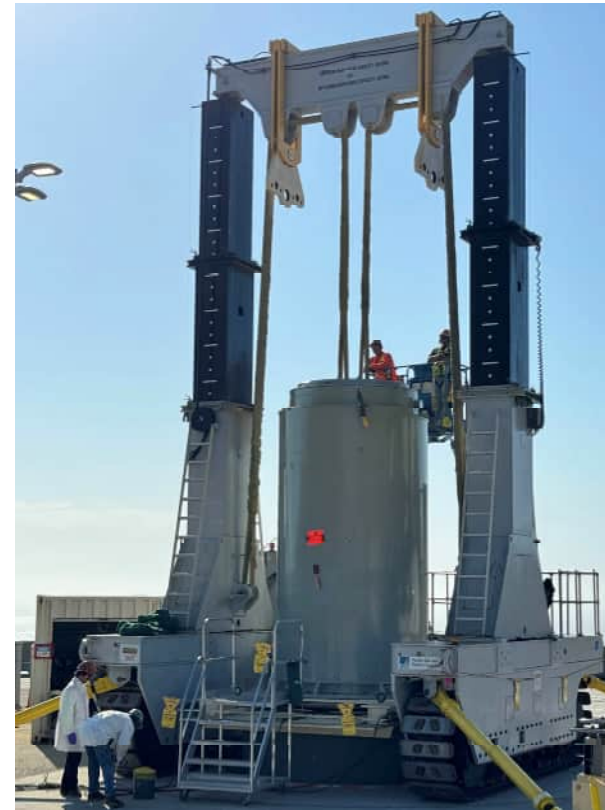
Transferring MPC from Transfer Cask (Hi-TRAC) to Storage Cask (Hi-STORM)
