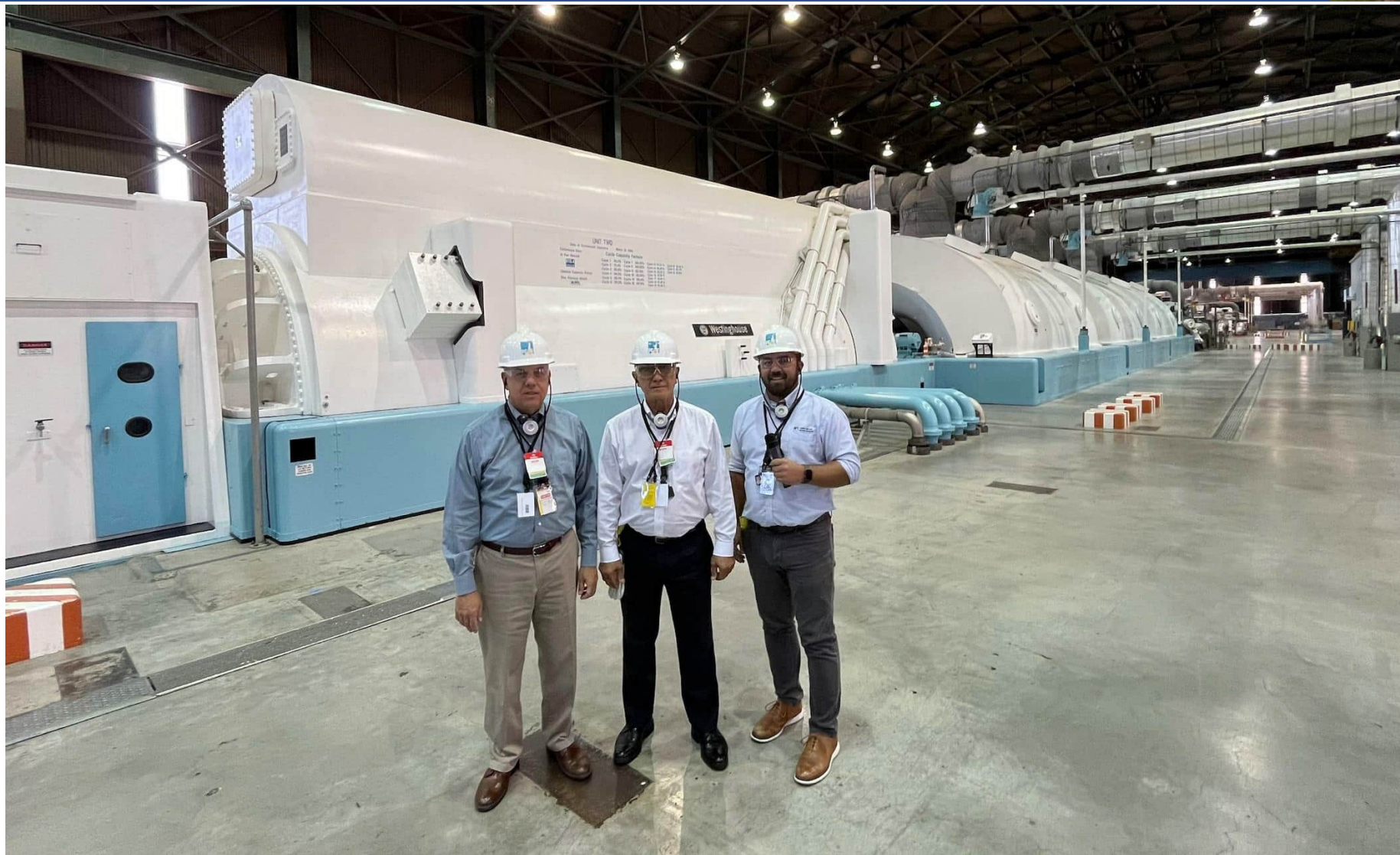
Fact-Finding Team On Turbine Deck
