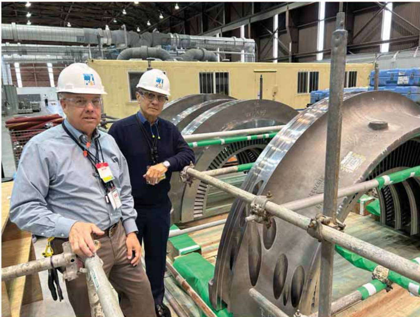
Mr. McWhorter and Dr. Meshkati at Replacement HP Turbine Stator Elements
