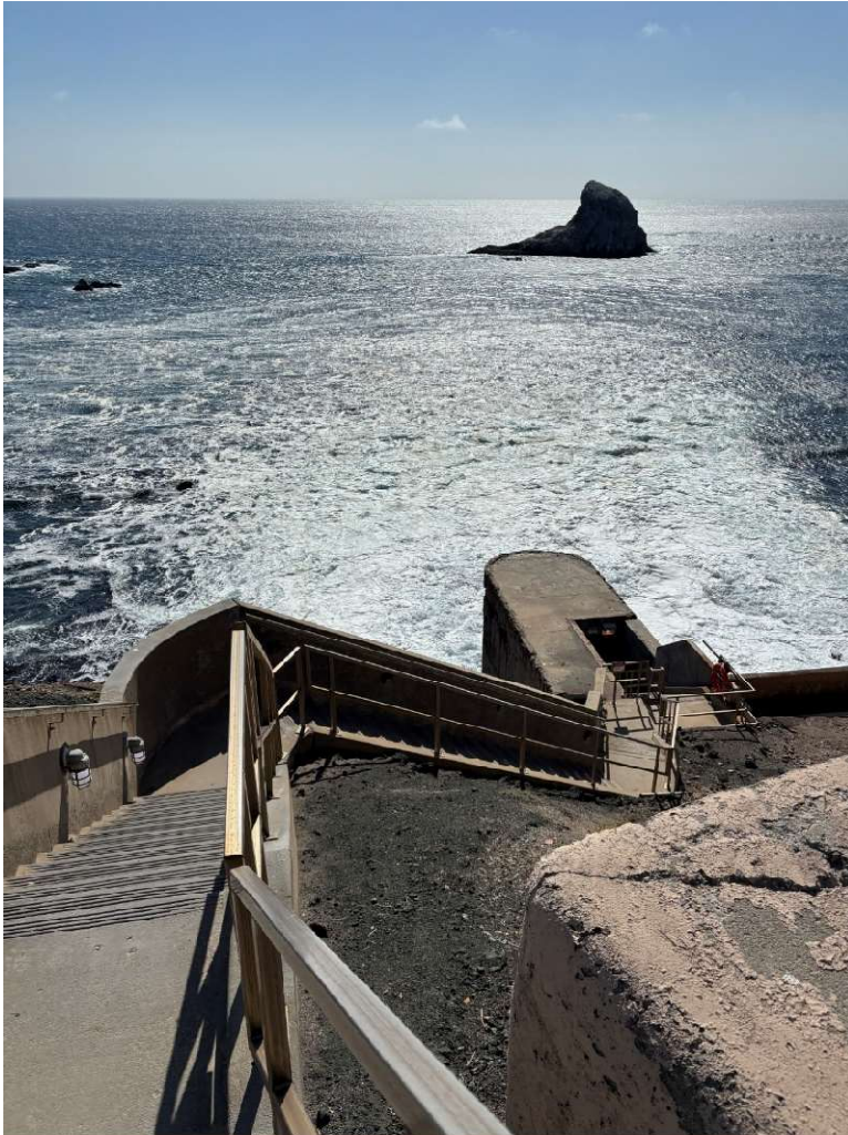
Access Stairway to Discharge Structure
