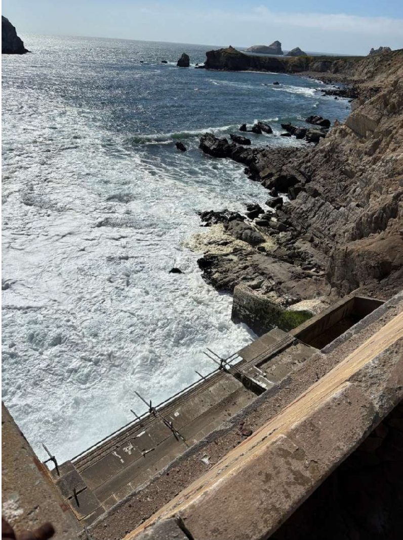
Discharge Structure Viewed from Access Stairway
