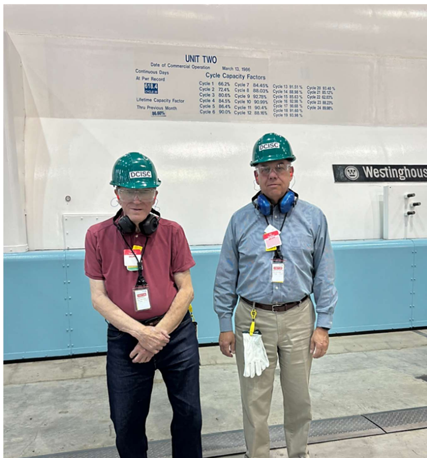
Dr. Budnitz and Mr. McWhorter at Unit 2 Main Generator
