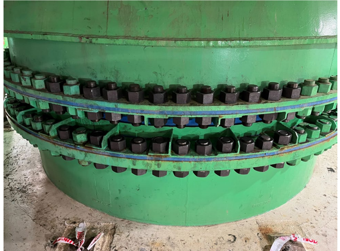
Condenser Saltwater E.J. Replacement (12ft dia)
