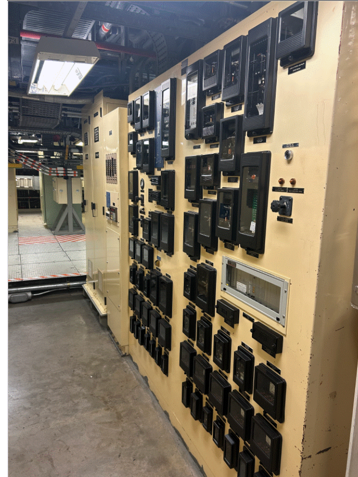
Main Generator Relay Replacement (21 EM to 6 Digital)
