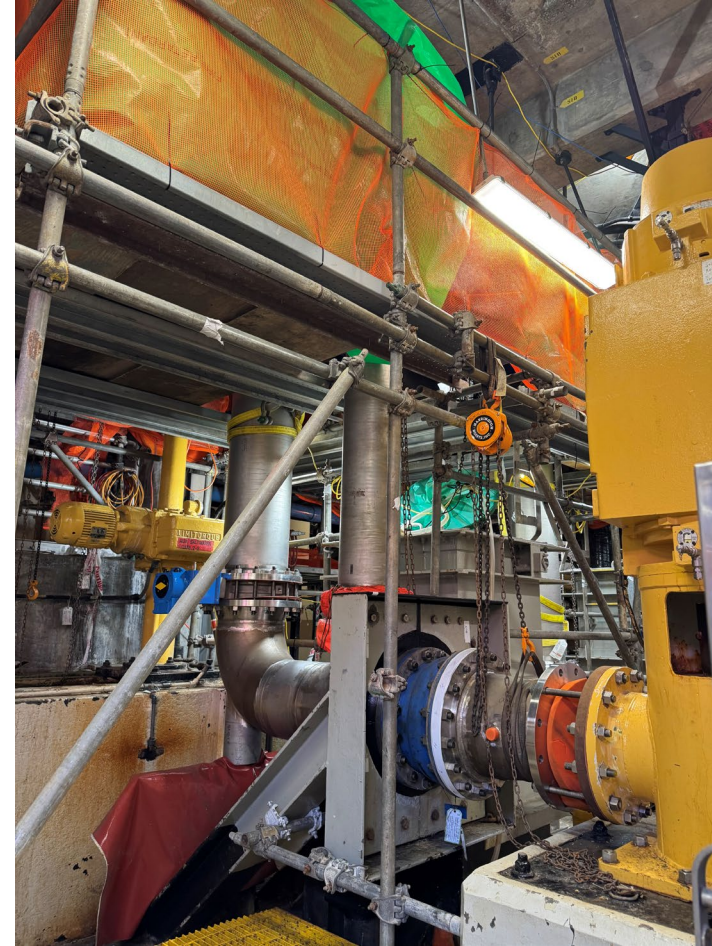
Intake Screen Wash Piping System Replacement
