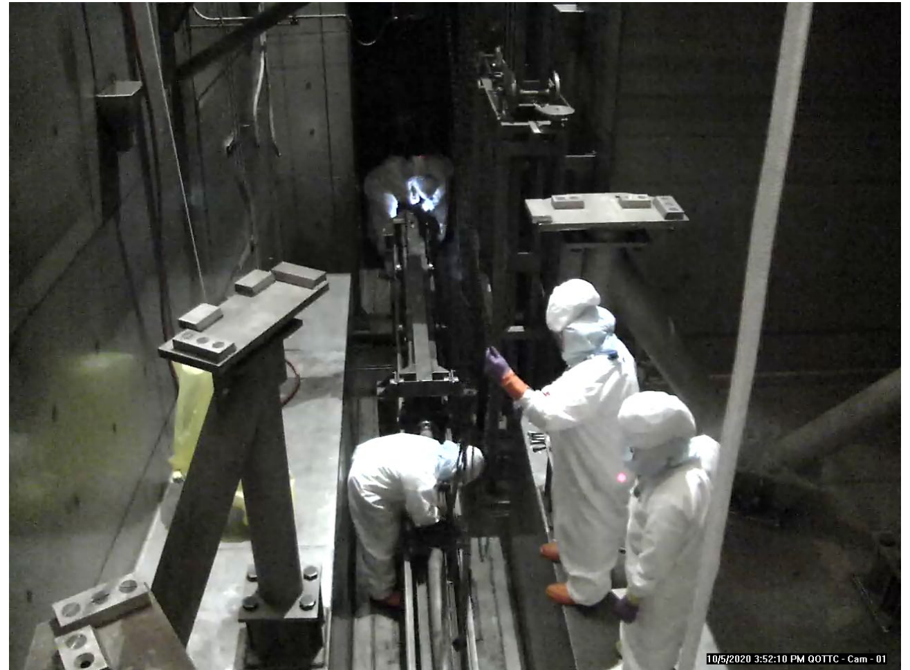
Fuel Transfer System Replacement
