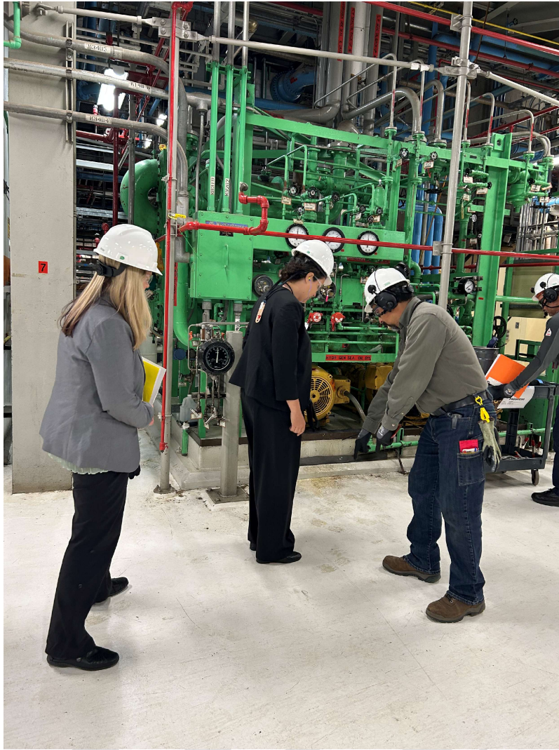
Ms. Darden, Dr. Scarlat, and PG&E I&C Technicians at the Unit 1 Air Side Seal Oil System.
